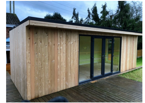
Leisure room 7m x 3m
